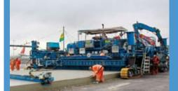
Wirtgen's slipform paver SP 1600 easily met the high quality demands at Amsterdam Airport, which specified a maximum tolerance of 5 mm over a length of 3 m in both longitudinal and transverse direction.
