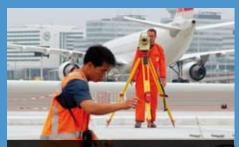
Verification measurements during the paving operation showed that the SP 160 worked with maximum precision: level and slope of the concrete surface precisely matched the specified requirements.
