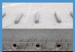
Dowel bars are inserted to ensure the bond between the 10m wide concrete slabs.
